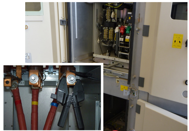
DLRO100 testing circuit breaker
